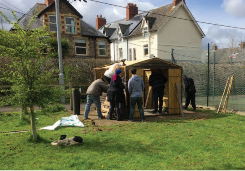
Seeds of Hope erecting a garden shed at their Watchet site
